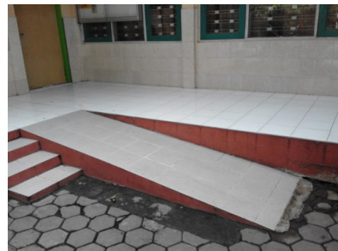
Figure 3. Ramp without handrails in School "A"
