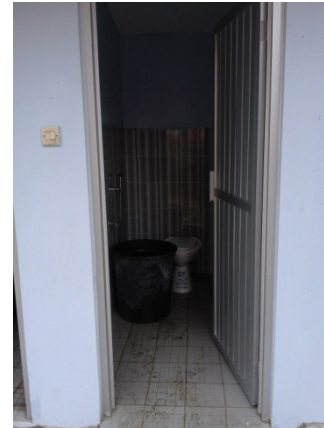
Figure 5. Toilet for children with special needs in School "A"
