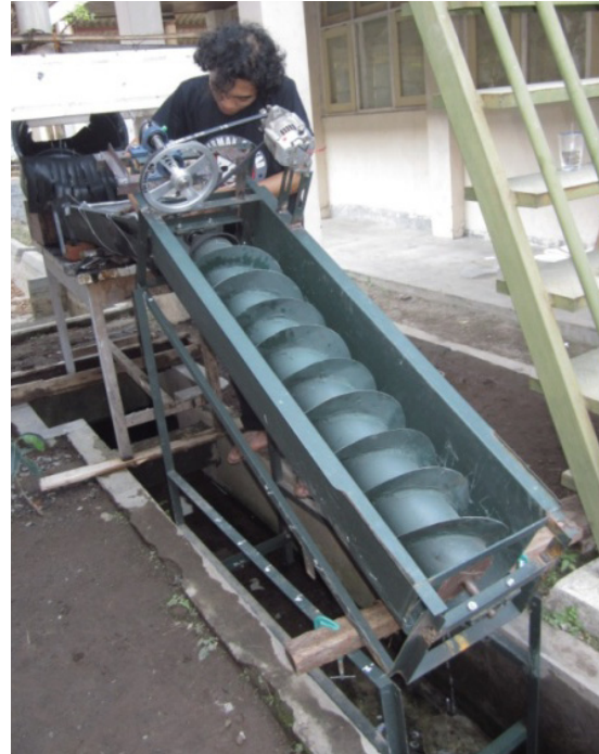
Figure 2. Installation of Screw Turbine
