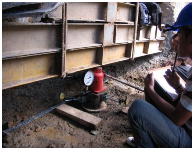
Figure 1. Obtaining Modulus Subgrade of Reaction using Plate Loading Test.
