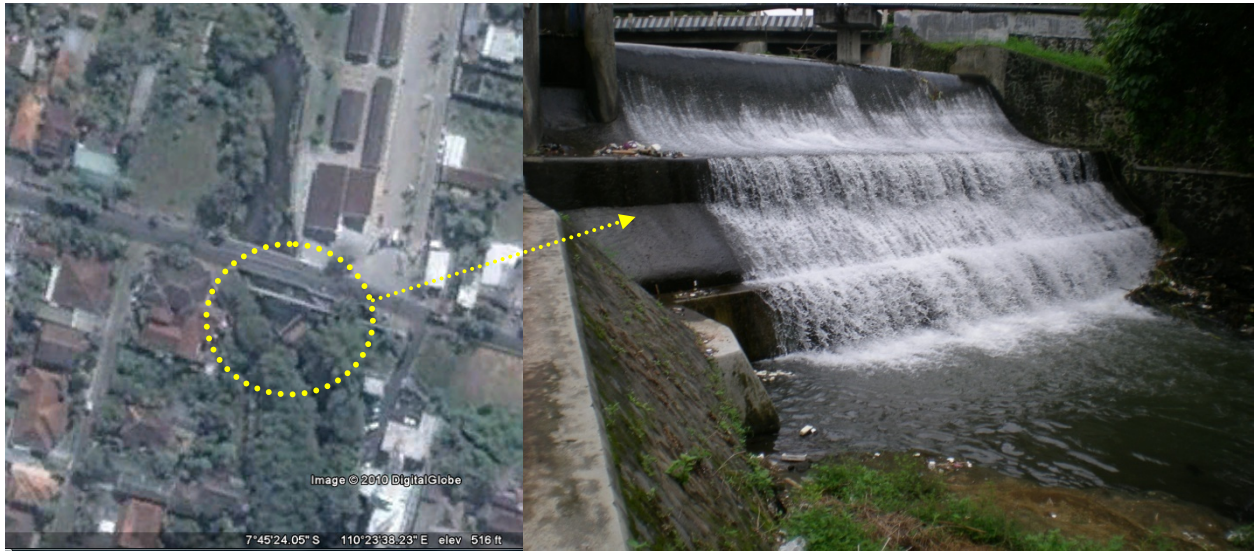
Figure 1. Cascade Weir at Gajah Wong River, Yogyakarta (The right picture was documented on 11 April 2010)
