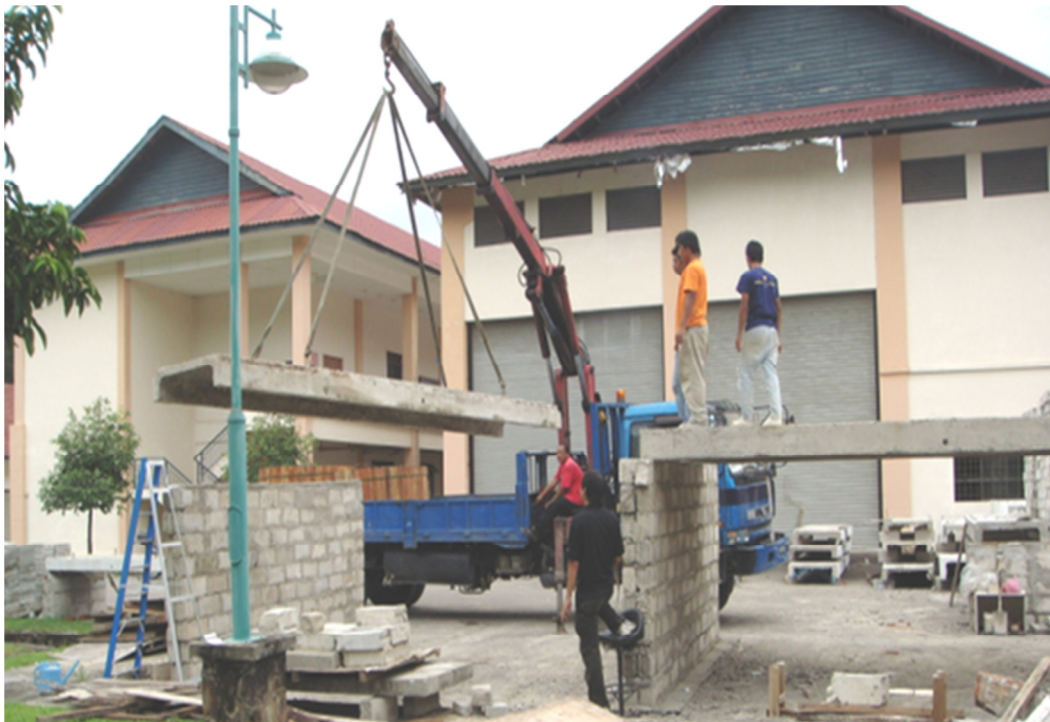
Figure 6: Erecting of C-channel using lorry mounted crane
