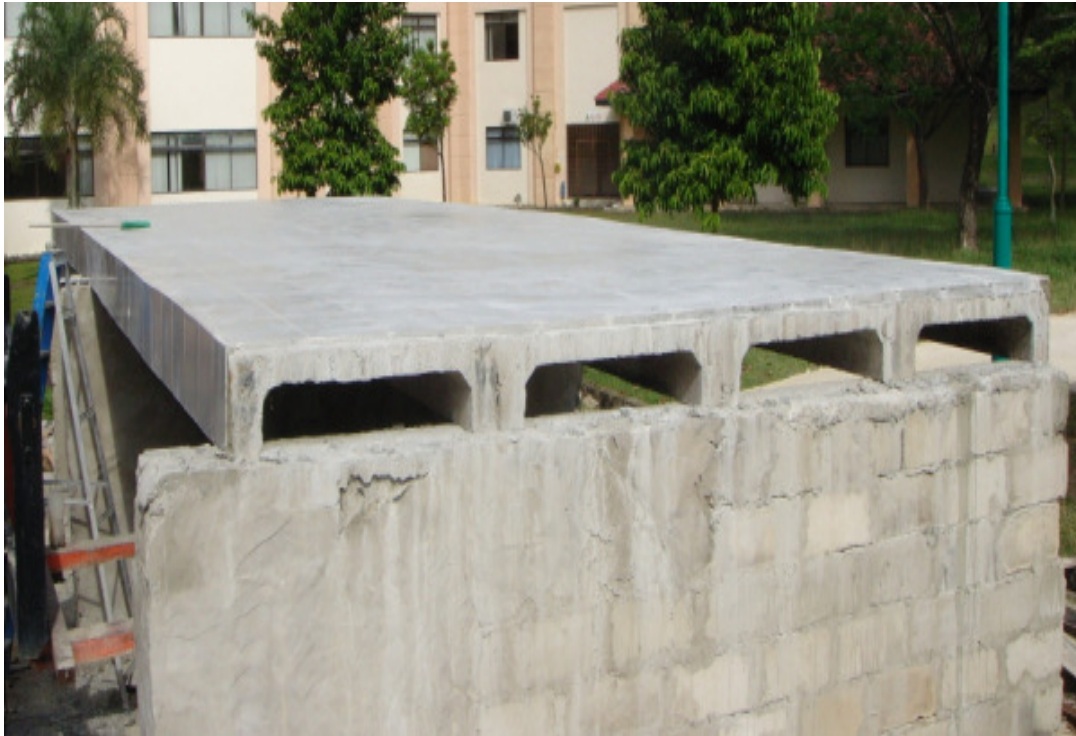
Figure 7: Completed C-channel floor structure with tile finishing
