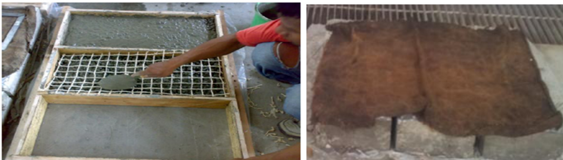
Figure 2 Sandwich Wall Casting and Curing Process
