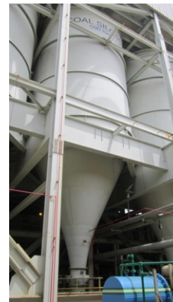
Fig. 1 Coal Silo Bunker.
